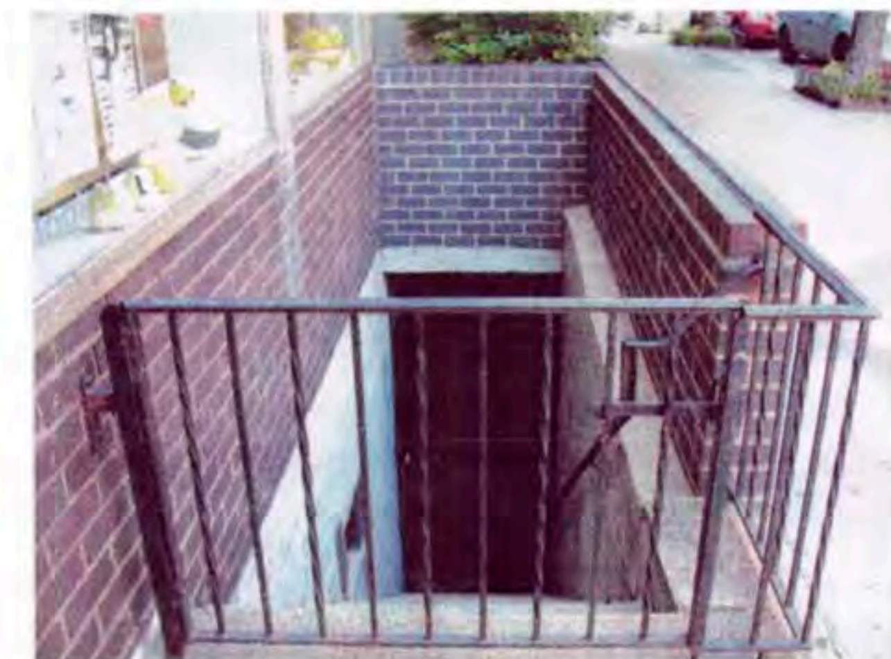
EXISTING STAIR AT BLEECKER STREET
