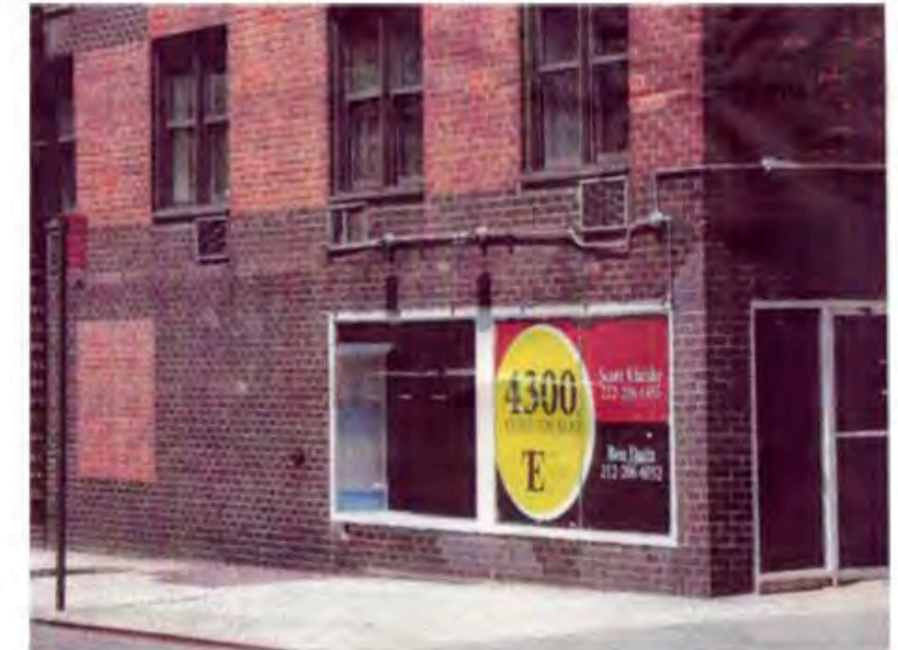
EXISTING FACADE AT WEST 10TH STREET
