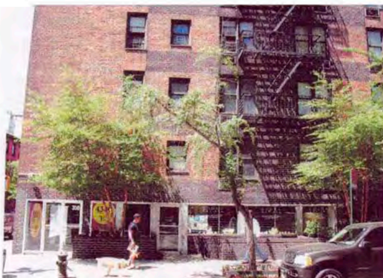
EXISTING FACADE AT BLEECKER STREET
