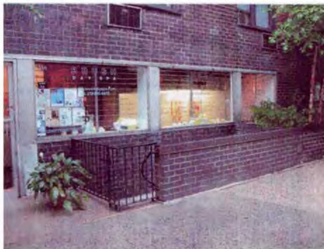
EXISTING STAIR AT BLEECKER STREET
